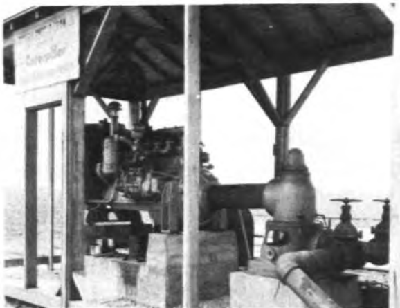
FIGURE 13. 1000 GALLONS-PER-MINUTE IRRIGATION PUMP AND DIESEL ENGINE INSTALLATION NEAR EL PASO, ILLINOIS.
